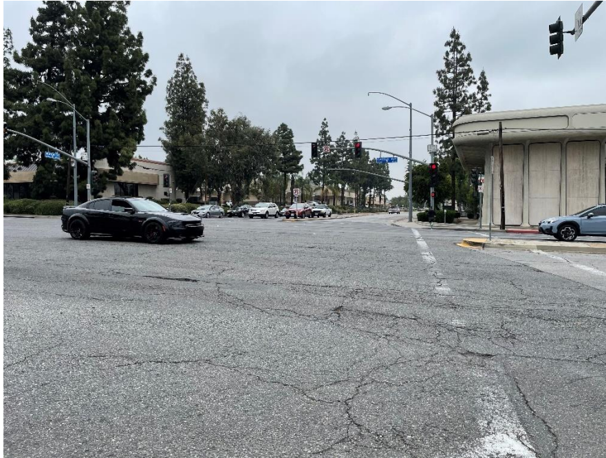
A faded crosswalk across Central Avenue, which decreases visibility of the pedestrian right-of-way
