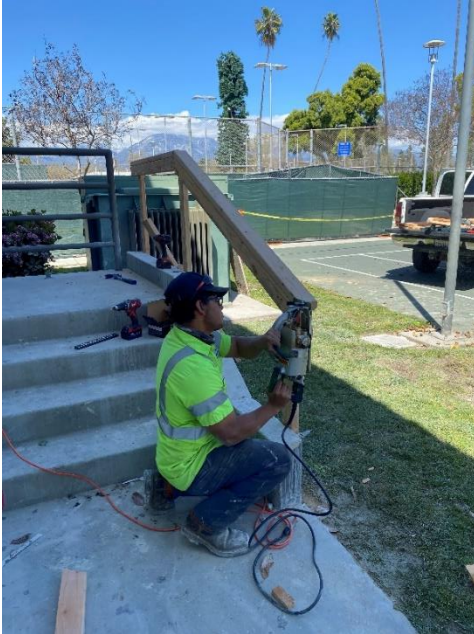
Maintenance worker Jose Rodriguez installing the new tubular rail and removing the temporary wood railing
