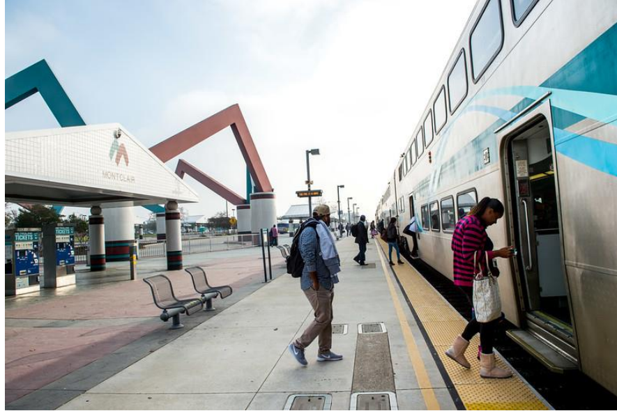
Passengers board Metrolink train at Montclair TransCenter. The boarding platform and rail line for the A-Line would be located along the visible area where the existing canopy structures and ticket booths currently exist.
