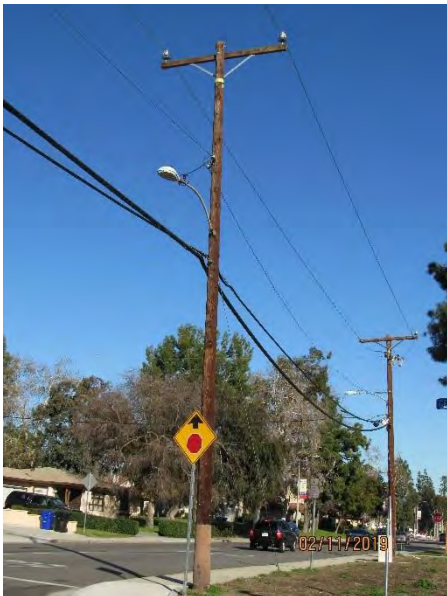
Non-Ornamental Transmission Wood Light Pole
