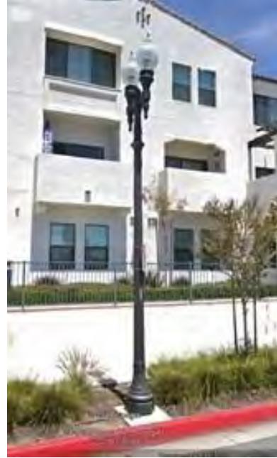
Ornamental Street Light Pole
