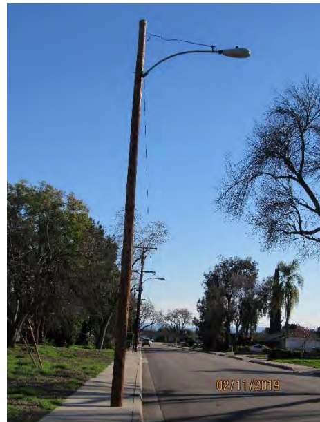
Non-Ornamental Distribution Wood Light Pole
