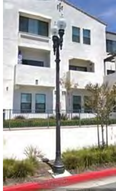
Ornamental Street Light Pole
