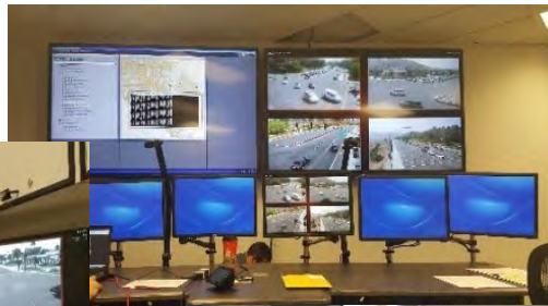
Santa Ana TMC under construction
