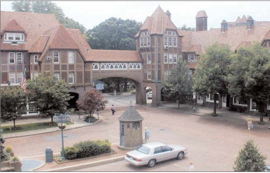
Great Station and Square: Forest Hills Gardens, Queens NY
