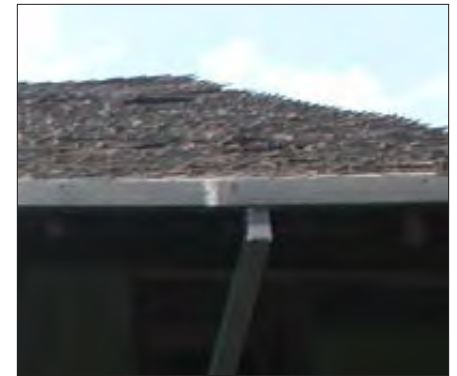
Gutter and downspout
