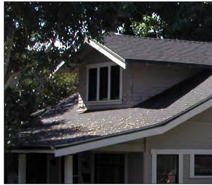
Dormer window with pitched roof
