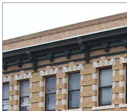
Parapet and cornice
