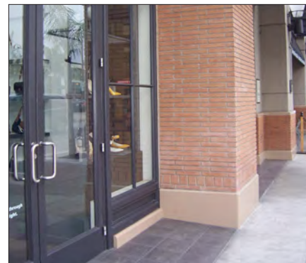
Concrete base with brick columns and walls
