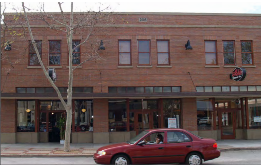
A Main Street Commercial style building with ground floor storefronts and upper floor double-hung windows grouped in threes.
