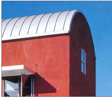
Metal barrel roof
