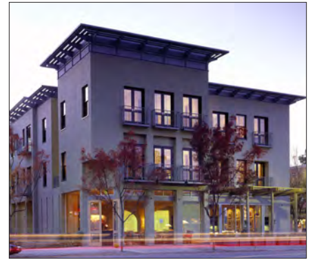
Flat roof with decorative parapet
