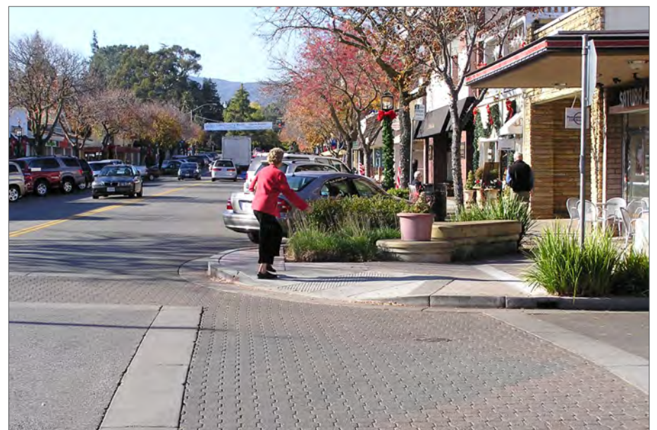
Crosswalks finished with pavers and cast concrete borders lead to a landscaped corner curb extension.
