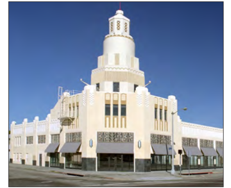
Corner stepped tower
