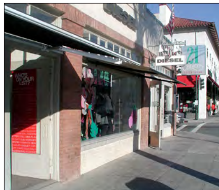
Painted brick transom
