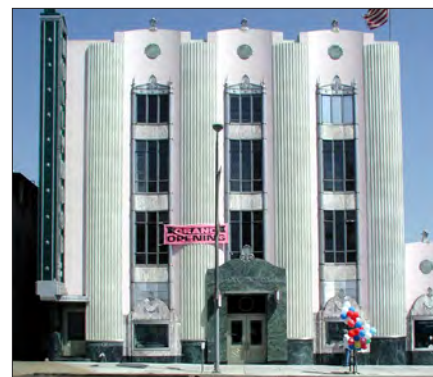
Plaster and metal
