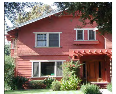
Painted shingles above painted lap siding
