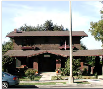
Roofs parallel to street
