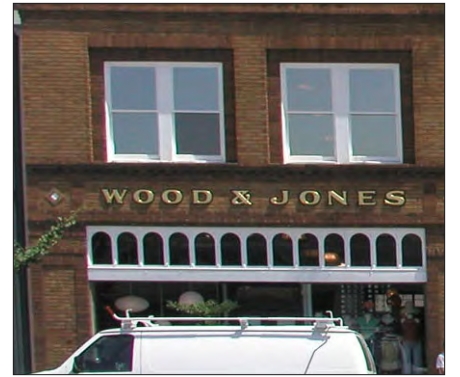
Articulated parapet with integrated signage
