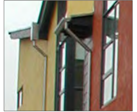
Scuppers and downspouts
