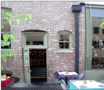
Downspout on back side of building;
