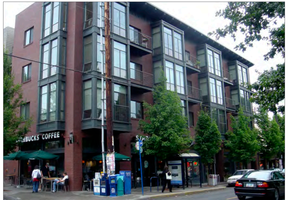
Three-story bay windows and balconies project from the facade of this mixed-use building.
