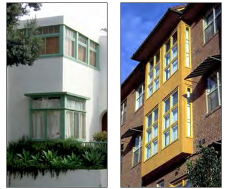
Corner windows, Bay Window
