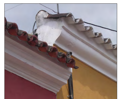
tile on profiled parapet
