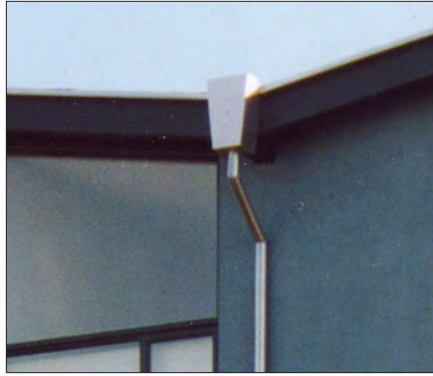
Scupper and downspout
