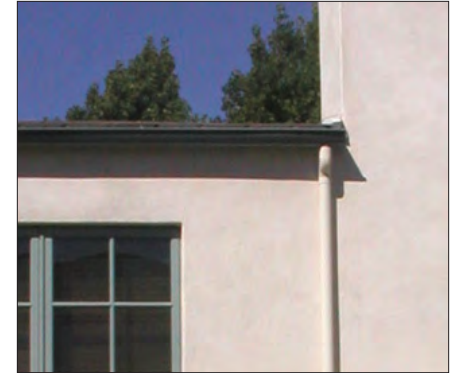
gutter and downspout
