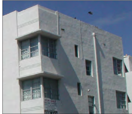
Scupper and downspout on building side
