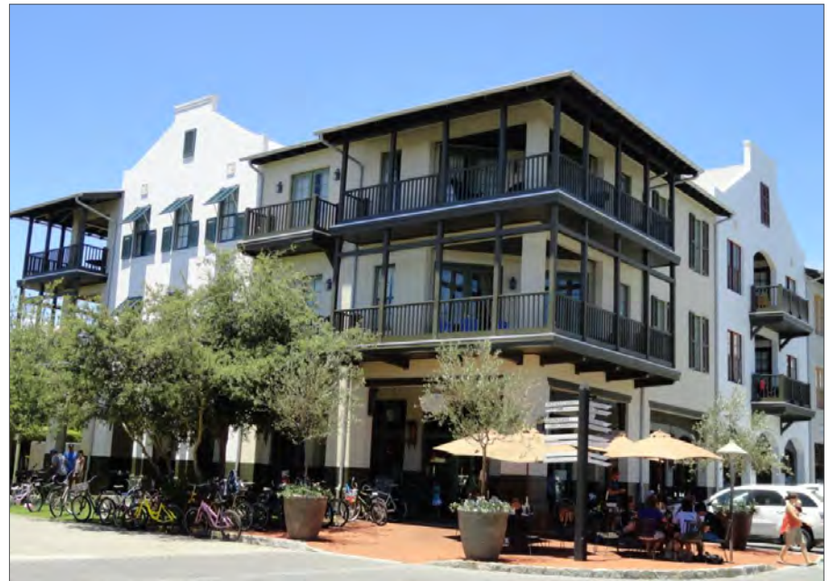
Upper floor balconies project from this mixed-use building.
