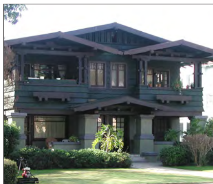
Siding above painted plaster
