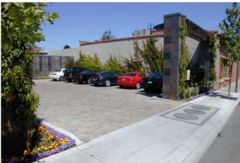
A commercial parking lot that includes planting areas and semi-permeable paving to facilitate rainwater recharging.
