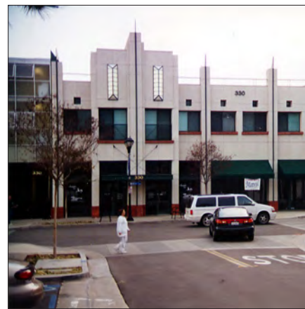
Terminated Street Vista
