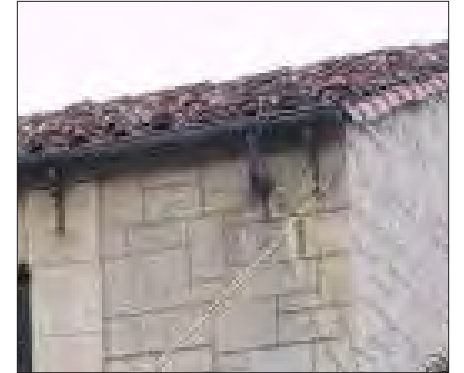
Gutter with downspout into wall
