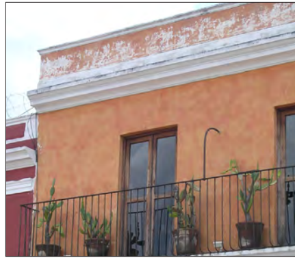
parapet with flat roof
