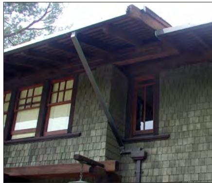
Gutter and downspout
