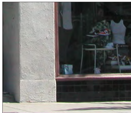
monolithic wall and base
