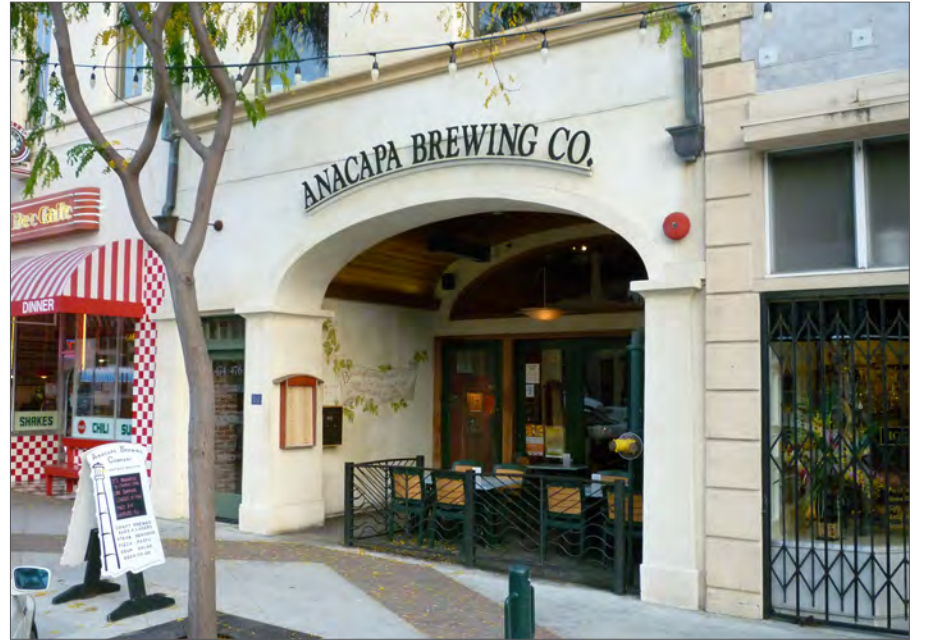
A recessed storefront accommodates covered, outdoor seating.
