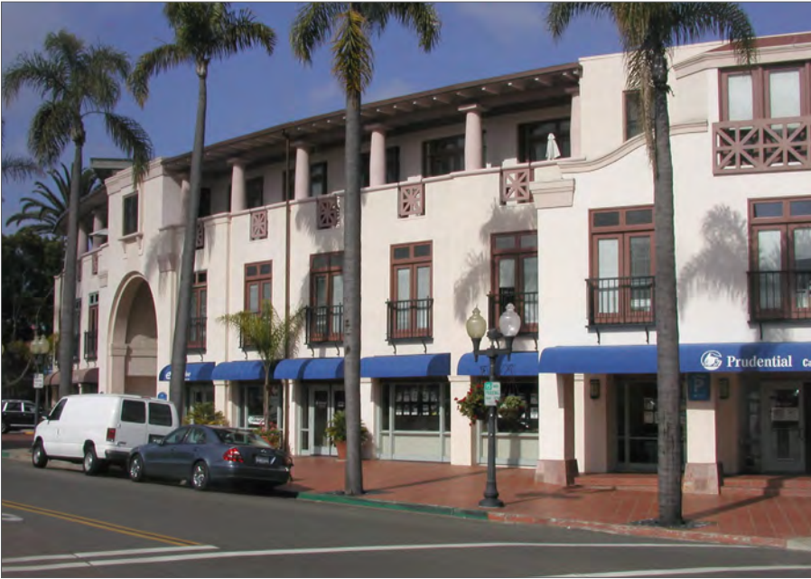
A third-story covered balcony, along with second floor French balconies help articulate this three-story mixed-use building.
