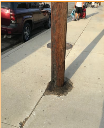
Utility pole in the middle of the sidewalk that presents barriers to pedestrians on wheelchairs or with strollers
