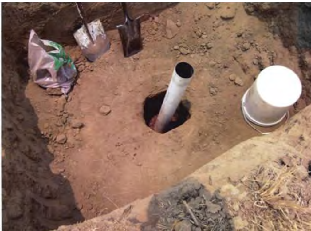
Figure VII.17. Photo of Percolation Test Pit.
