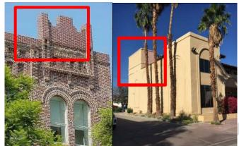
**Roof-mounted facilities** shall be screened from view by a treatment that compliments the architecture of the building or structure, or be designed to be visually integrated with the host structure.
