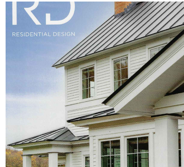
STANDING SEAM METAL ROOF MEDIUM GRAY APPROXIMATE
