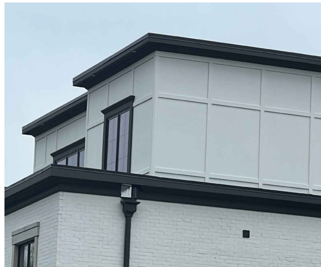
HARDI MATERIAL (TRIM & BOARD) REF. TABLE ABOVE FOR COLOR (SWISS COFFEE)
