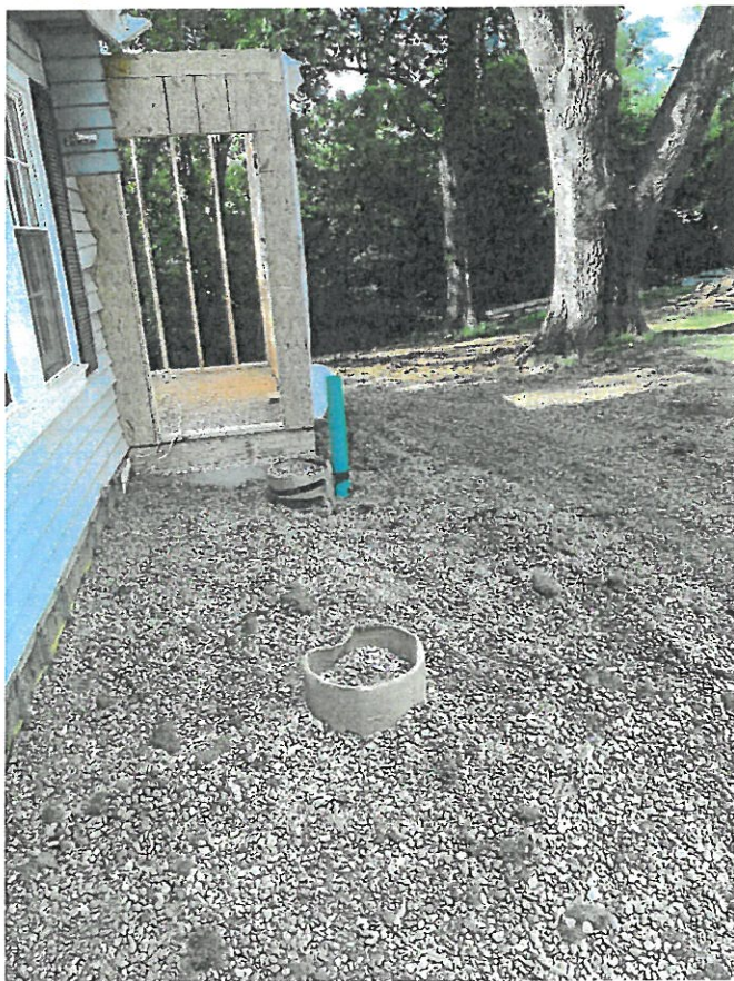
EAST WALL BACKFILLED WITH 100% GRAVEL AND (2) LAYERS DRAIN TILE (HIDDEN FROM VIEW)
