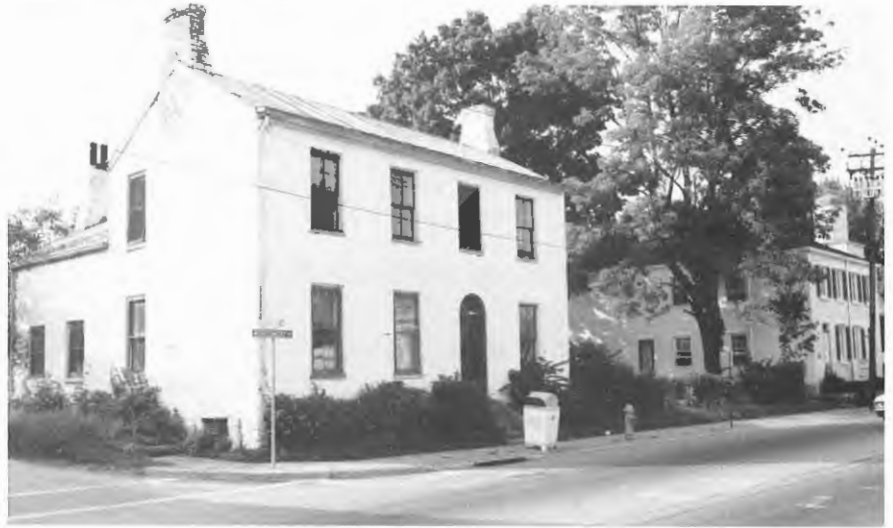
Presbyterian manse c. 1820s which was razed in 1971 for Montgomery Cyclery.
