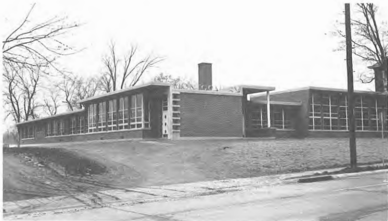
A photo taken in 1952 of the just-completed Montgomery Elementary School.
