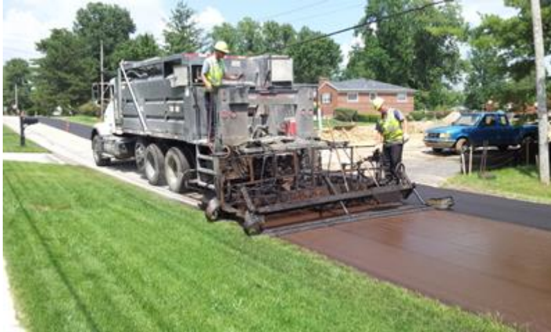
Roadway Repaving Project
