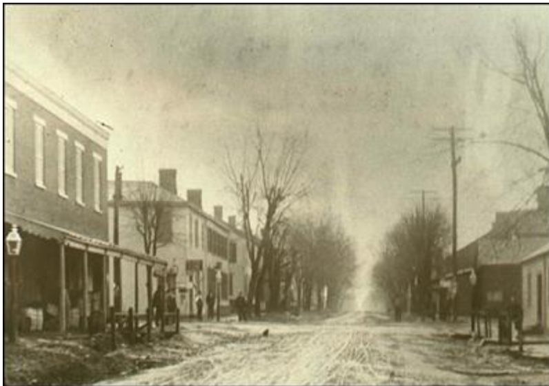
Montgomery Road before it was paved
