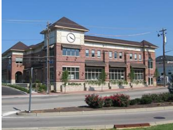
Montgomery Center East
