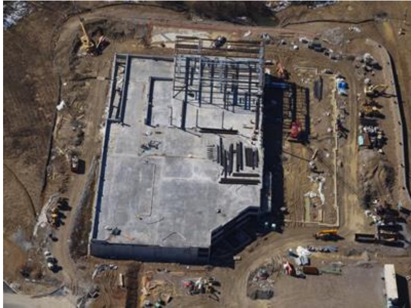
Aerial shot of Christ Hospital construction site
