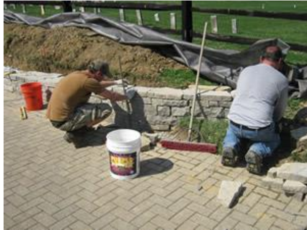
Installation of new stone wall at Hopewell Cemetery
