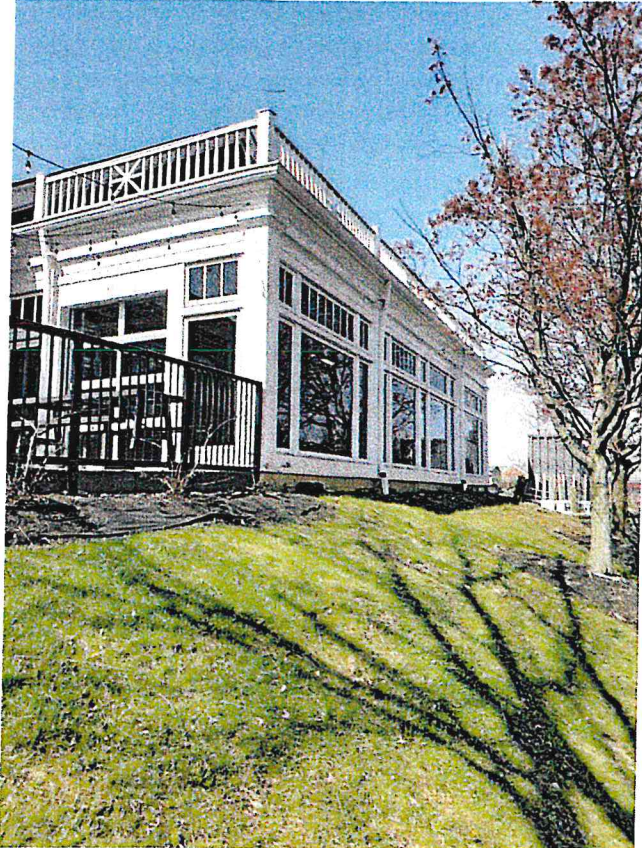
Deck Location, looking north up Main Street
