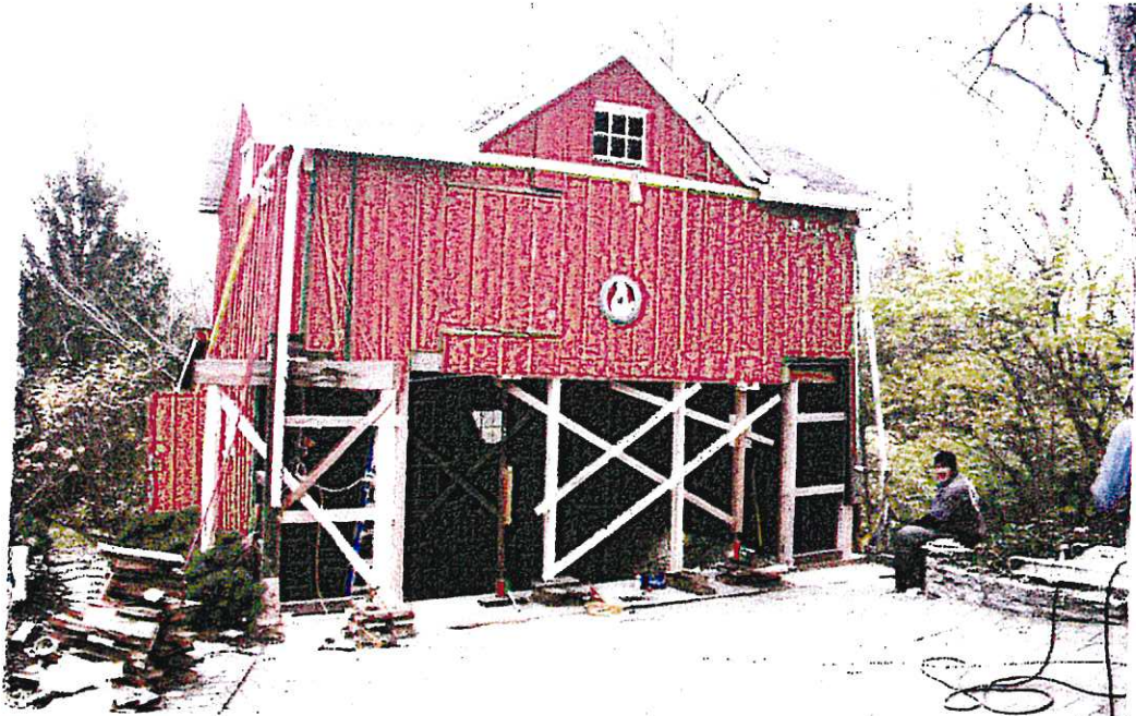
View of barn, north-facing front elevation
