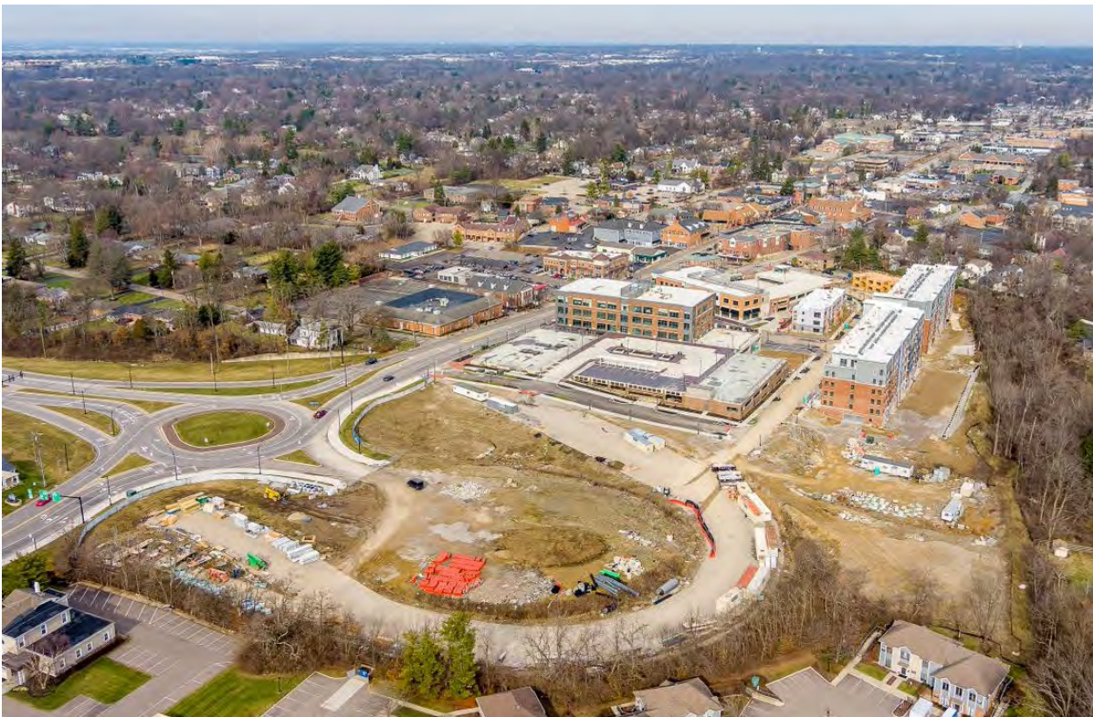
Phase 2 area looking North.
