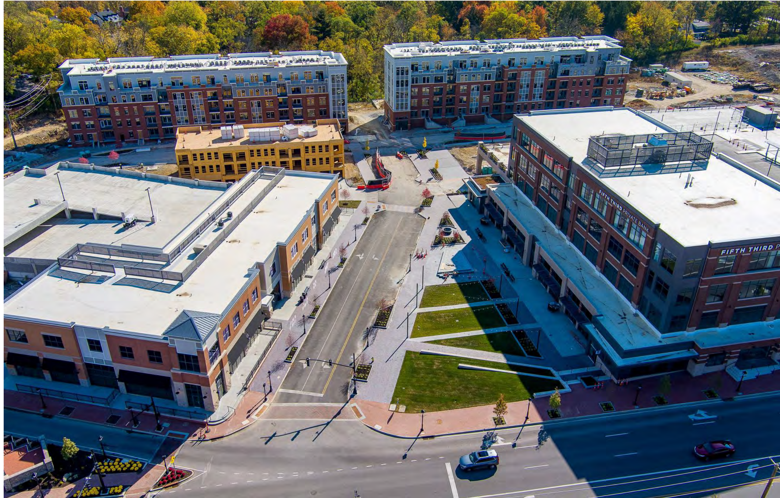
MQ - Phase 1 Drone Photo - October 2022
