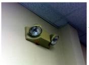
Emergency light fixtures are equipped with a test button. Pressing the test button simulates a power failure enabling the battery to power the white flood lights as shown in this picture. If they do not come on, come on dimly, or hum then the fixture probably needs a new battery.
