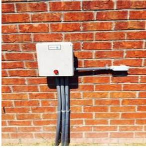
Many City of Munford sewer customers rely on a "STEP sewer system" to discharge household wastewater to Munford's city-wide sewer system. "STEP" stands for "Septic Tank Effluent Pump" and these systems are used throughout the United States. If you are one of our STEP customers, it's important that you are aware of that fact, and understand how it works at your location.
