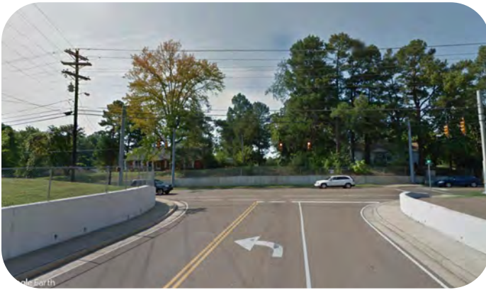
NARROW SIDEWALKS ALONG STREET EDGE
