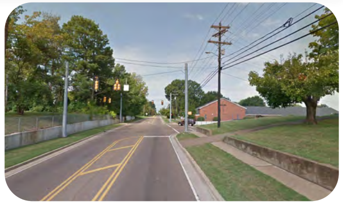
EXCESSIVE LANE WIDTH
