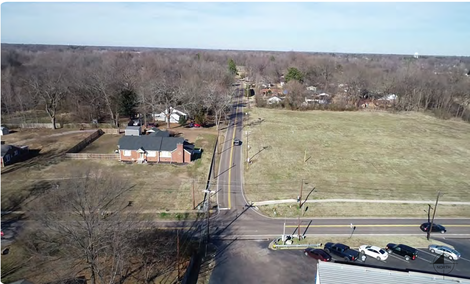
LOOKING NORTH AT THE INTERSECTION OF MAIN STREET AND GILTEDGE ROAD.
