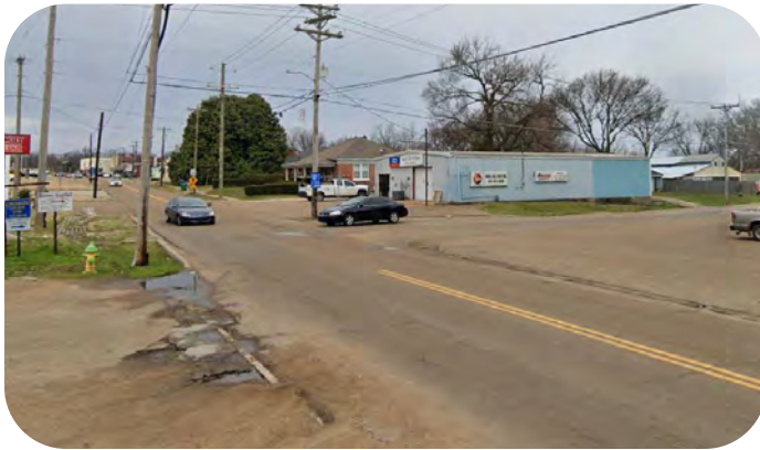
DRAINAGE IMPROVEMENTS NEEDED
