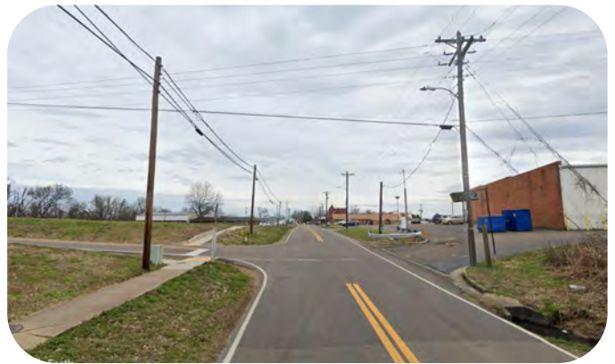
UTILITY LINES ALONG MAIN STREET
