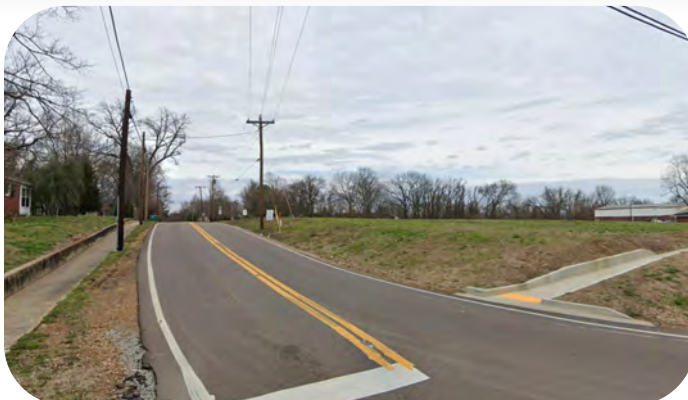
LACK OF SIDEWALKS ON EAST SIDE OF GILT EDGE RD
