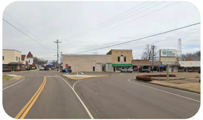
EXCESSIVE ASPHALT ON TIPTON STREET
