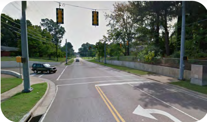
CROSSING DOES NOT CONNECT TO A SIDEWALK
