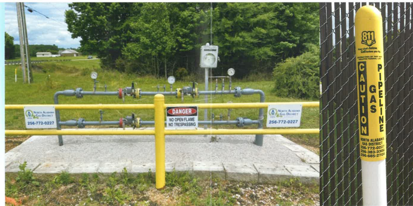
Pipeline markers & flags identify the approximate location of underground pipeline facilities. Markers & flags also provide relevant contact information for North Alabama Gas District. Please do not destroy the markers & flags as they are there for a reason.
