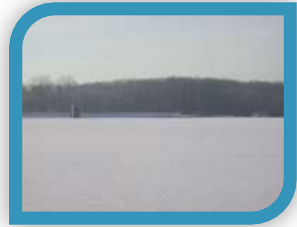
Lake Intake and Spillway
