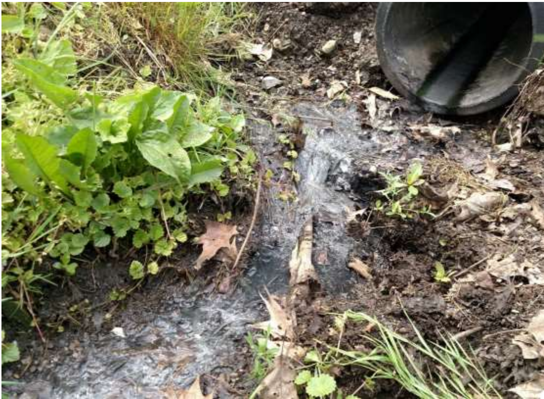
Figure 1: Raw sewage found in a ditch in North Lawrence
