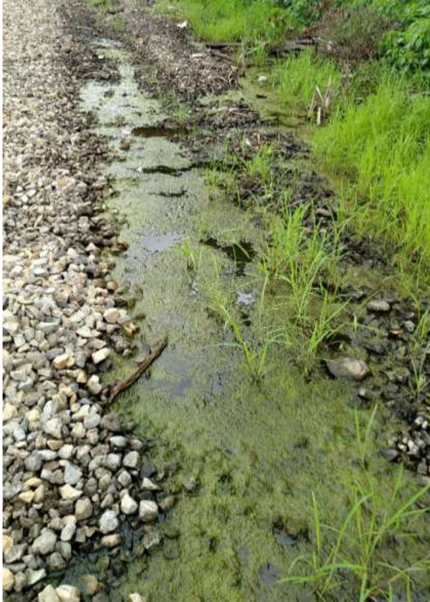
Figure 4: Ditch full of algae behind houses in Justus with failing septic systems.
