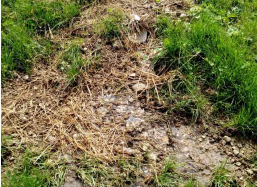
Figure 2: Water flowing over the ground as a result of flushing in a nearby house
