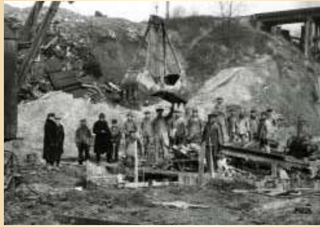
The combined sewer system under construction in the 1920s.
