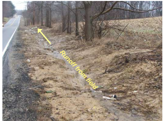
PI-105 Johnson Ditch at Mogadore Rd. Roadside ditch carrying sediment to Johnson ditch March, 2009.
