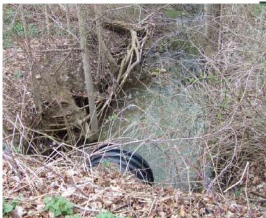
B-580 Breakneck headwater tributary, Wilkes Rd. (slope 2.3%) Banks are eroding. April, 2011.
