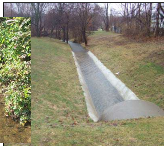
MS 280, 270 Kelsey Creek in Kennedy Park lacks a functional riparian corridor and is eroding its banks, partially due to excess stormwater from altered stream corridors and impervious surfaces in neighborhoods. The sediment and channel erosion degrade the stream habitat. Many streams in the Main Stem subwatershed are altered. Spring, 2011, Summer, 2010.
