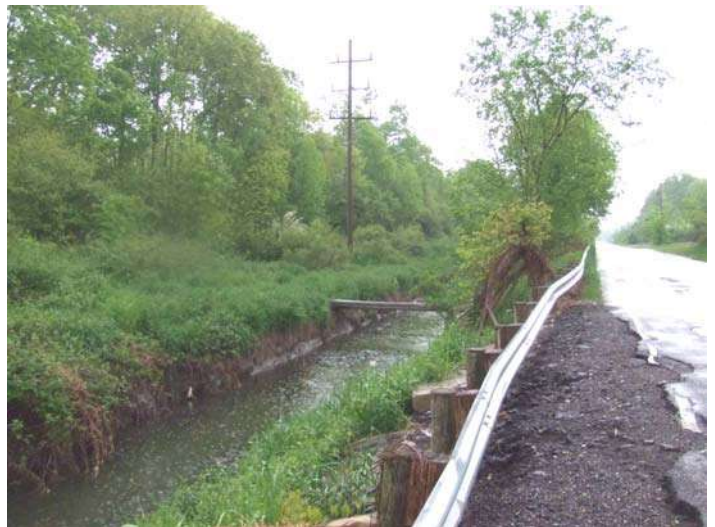
B-151; 156; 157. Hommon Ave. Ditch—(left) B-151—upstream of Ravenna Wastewater Treatment Plant; (lower left) B-156—downstream of wastewater treatment plant (WWTP in background right); and (below) B-157—where the bank and road appear to be eroding. Note high tension power lines in corridor, which would constrain channel reconstruction. May, 2011. Pics 25226, 30, 31
