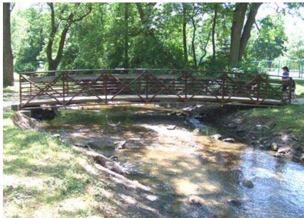
MS-300. Kelsey Creek in Water Works Park. The channel is gravelly. Erosion, which may be threatening the bridge, may be due to high volumes. June, 2011.
