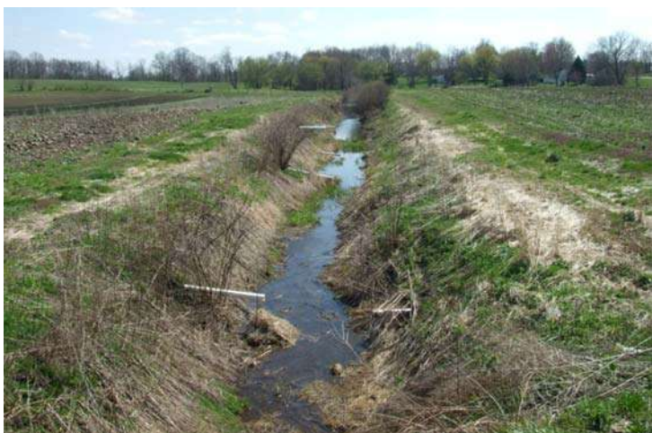
Po-370 Redinger Ditch at Alexander Rd. Grassed buffer. Tile outlets apparent. Spring 2011.
