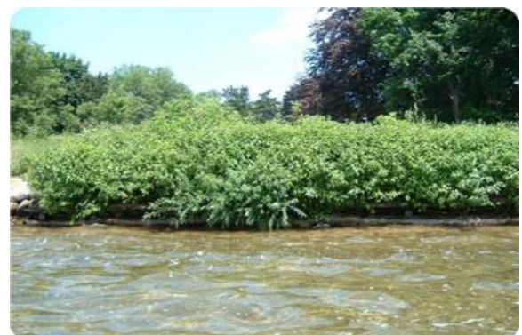
Live cribwall, summer 2005.
