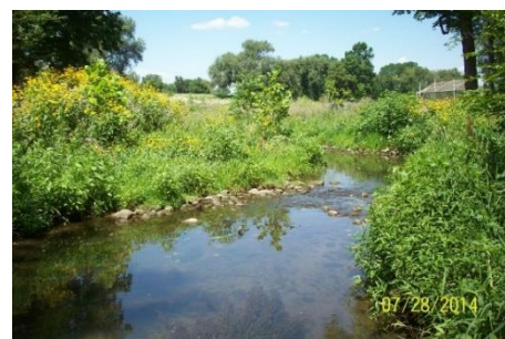
Formerly incised stream, with restored channel and floodplain. Photo source: R. McCleary, 2014.
