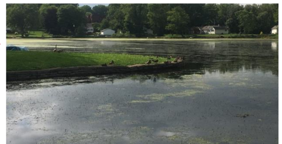
No 2 North Reservoir choked with vegetation, summer, 2020.
