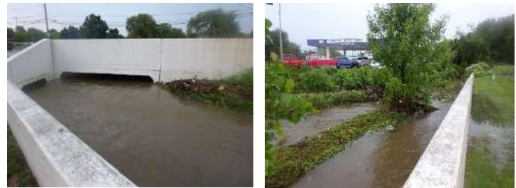
In highly altered Brewster Creek, a little extra room lets it spread out during high flow, reducing erosion, sediment transport, and downstream flooding. S. Main St.
