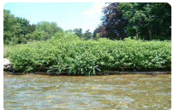
Live cribwall, summer 2005.
