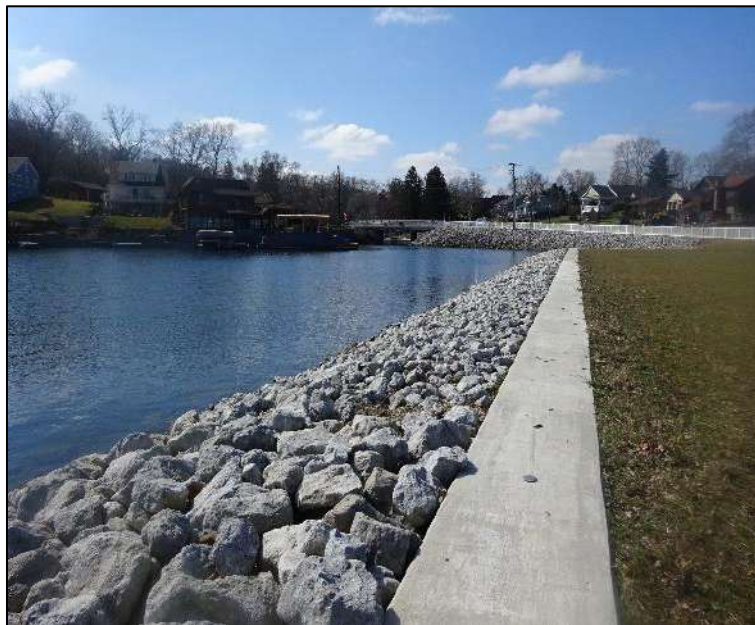
East Reservoir dam, 2020
