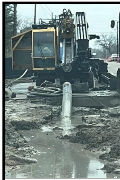
Roemer Utility Services Directional Drilling
