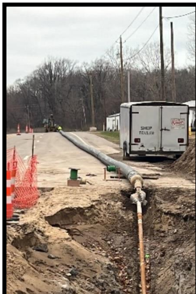
Sewer Force Main, Pre-pull
