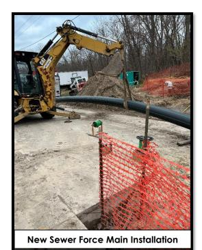
Last week, the sewer force main was relocated below US-12. Roemer Utility Services performed directional drilling of the force main successfully. This work was completed next to the boardwalk location, so that construction on the boardwalk can begin in the following weeks.
