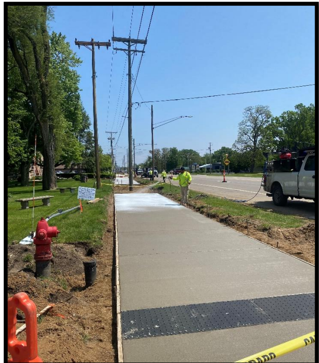
Curing Compound Sprayed on New 10 Foot Wide Non-motorized Trail
