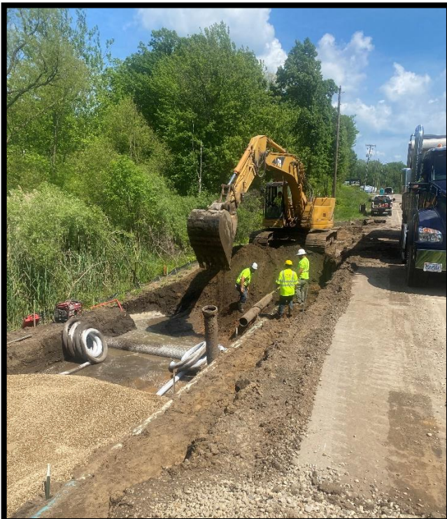
Construction of the Sub-grade Layer in Preparation for the Retaining Wall
