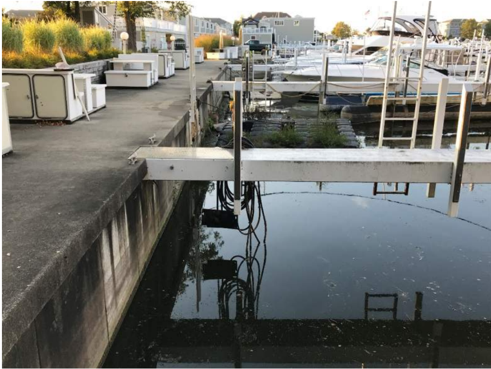
Seawall and Docks for SC1, SC3, SC5
