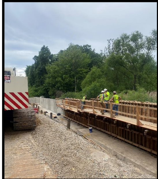
Anlaan Corporation Setting Retaining Wall Forms
