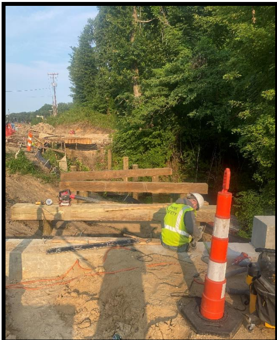
Beginning of Boardwalk Installation
