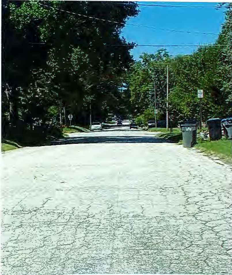
Michigan Street Reconstruction
