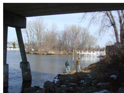
10 Under Whittaker Bridge looking west
