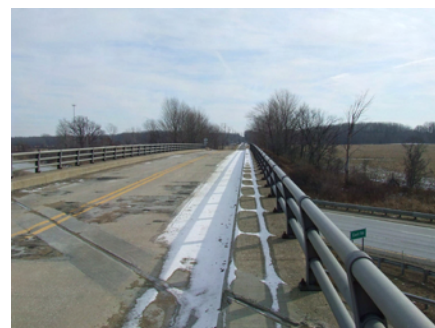
25 East at I-94 Bridge
