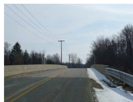
1 Maudlin @ 1-94 looking east
