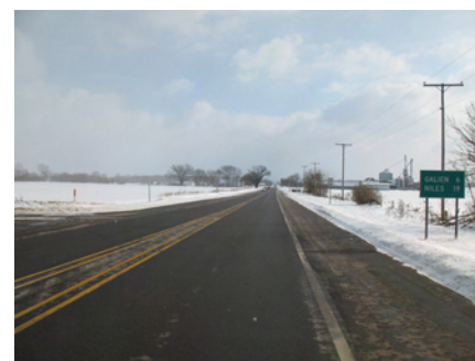
41 US-12 East of Three Oaks looking east
