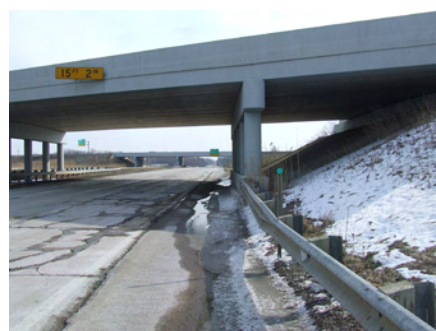
34 US-12 @ I-94 looking east
