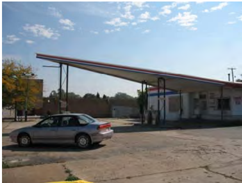
1960 era gas station, Benton Harbor
