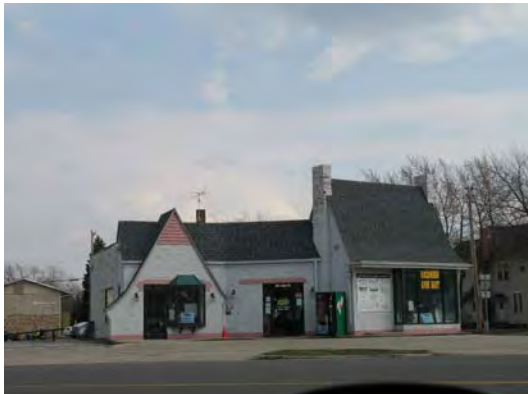
Red Arrow Highway, St. Joseph
