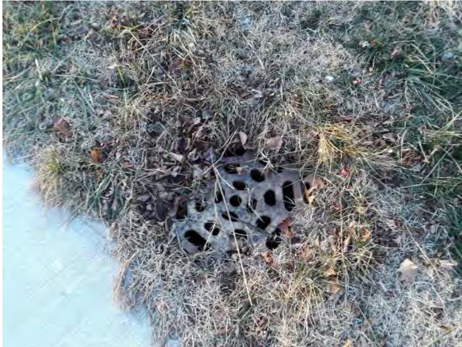
Image 7. Additional drainage structures located along W. Mechanic Street contributing to stormwater runoff and likely sediment loading.
