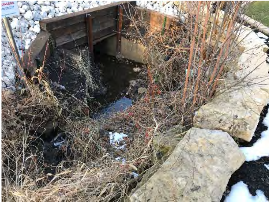
Image 5. Eroded soils and pollutants flow unimpeded into closed stormwater system
