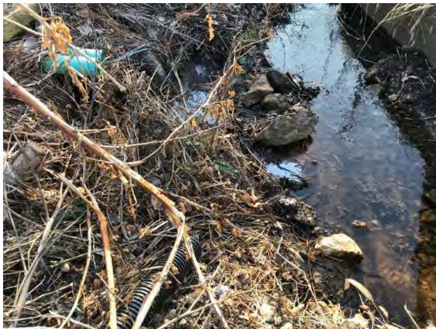
Image 6. Existing yard drains discharge directly into existing City stormwater system
