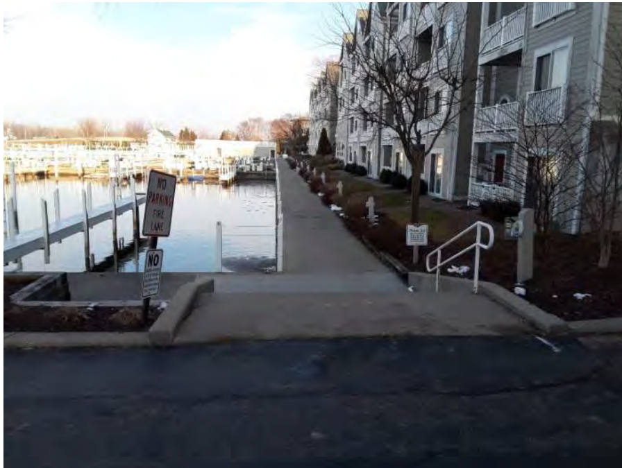
Image 2. City stormwater system outfall terminates at private mooring slip
