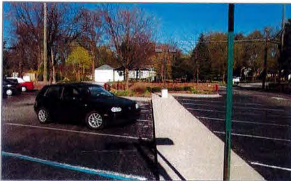
Parking lot with paved area between parking stalls for pedestrian circulation to minimize conflict with auto traffic
