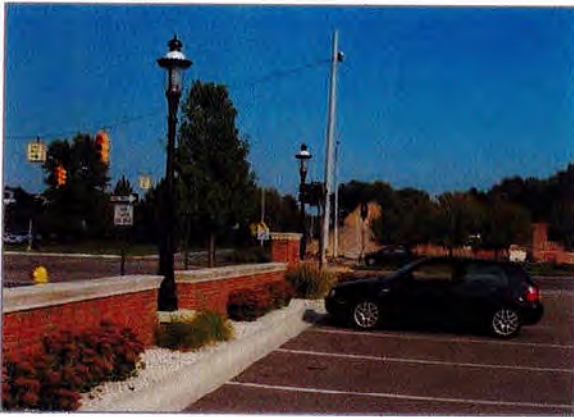
Parking lot with brick screen wall, perimeter pedestrian light fixture, landscaping strip and a raised concrete curb for a wheel stop
