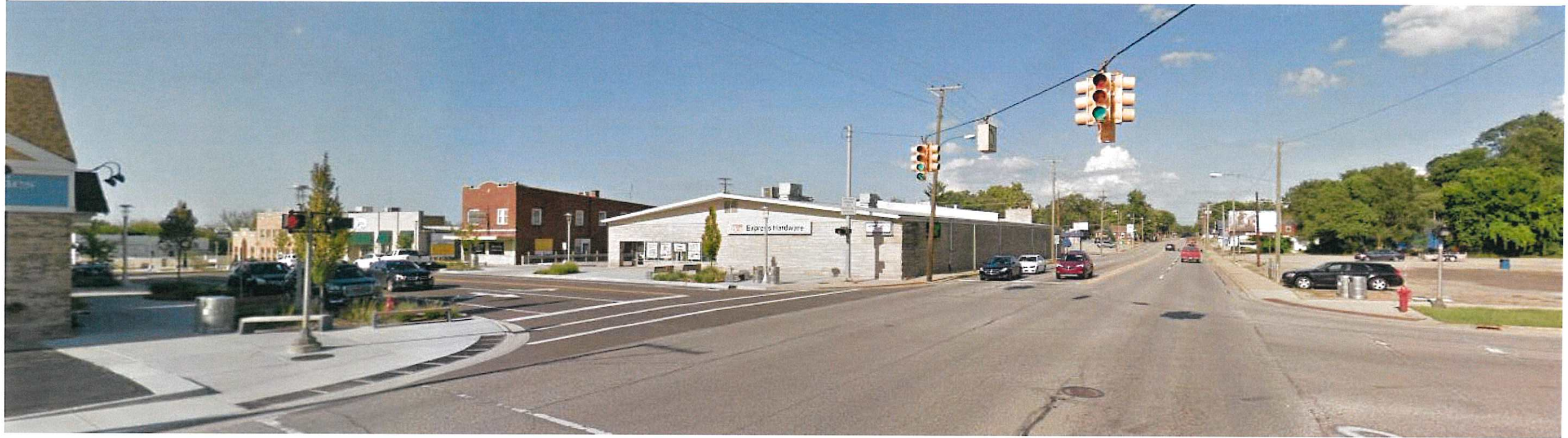
Existing Street View Looking Northeast
