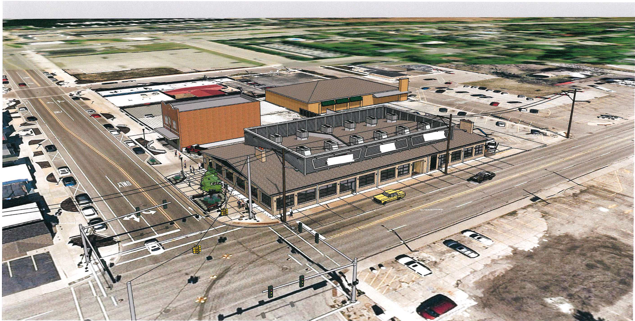
ARIAL CORNER VIEW
