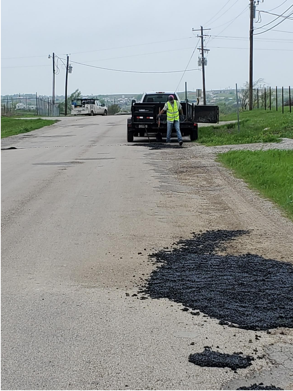
Jamie pothole patching on Hilltop Trail
