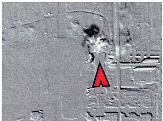
No. 12 Leak observed at an actuator on Separator L in High Sensitivity Mode.
