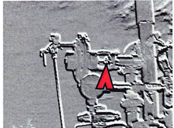
No. 2 Leak observed at a kimray valve on Well C in High Sensitivity Mode.
