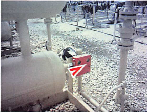
No. 9 Leak observed at an actuator on Separator F.
