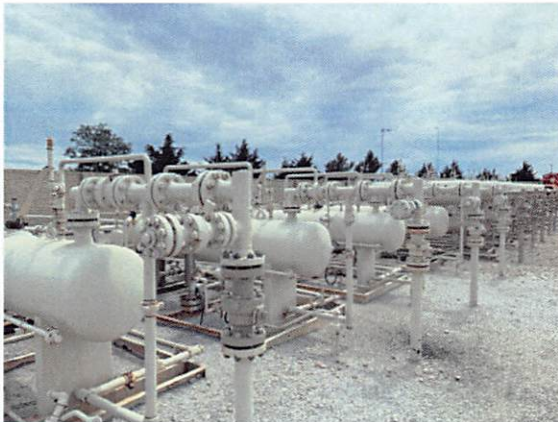
No. 15 View of separators.
