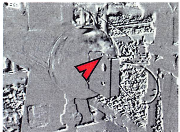
No. 6 Leak observed at an actuator on Separator B in High Sensitivity Mode.
