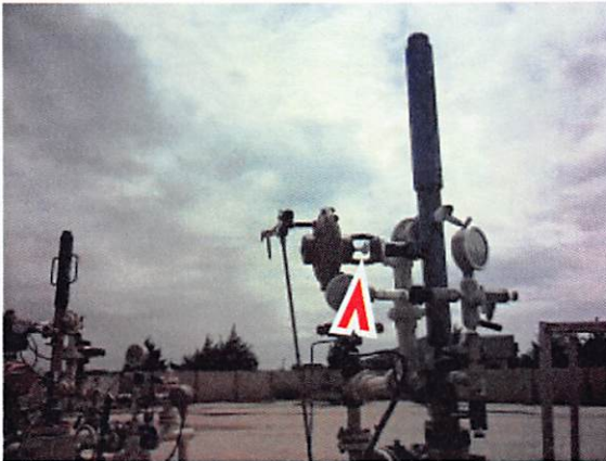
No. 1 Leak observed at a kimray valve on Well C.
