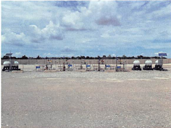
No. 13 View of wells.
