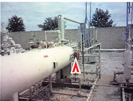
No. 11 Leak observed at an actuator on Separator L.
