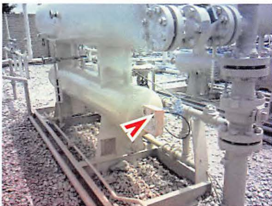
No. 5 Leak observed at an actuator on Separator B.
