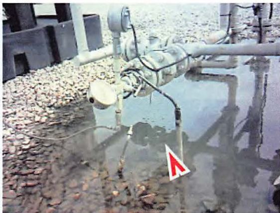
No. 3 Leak observed at a subgrade leak (bubbling) on Well L.
