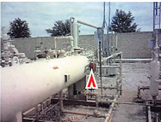
No. 11 Leak observed at an actuator on Separator L.
