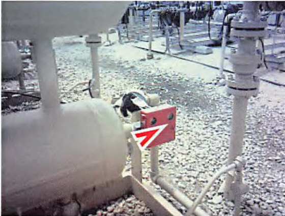
No. 9 Leak observed at an actuator on Separator F.
