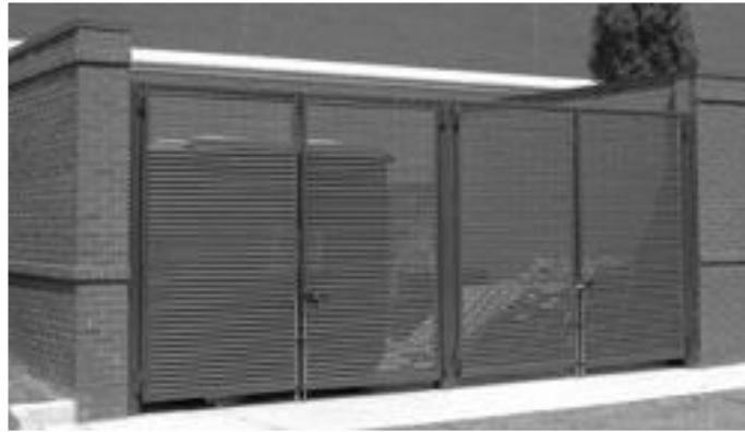
Masonry Refuse Container Enclosure (With Gates)
