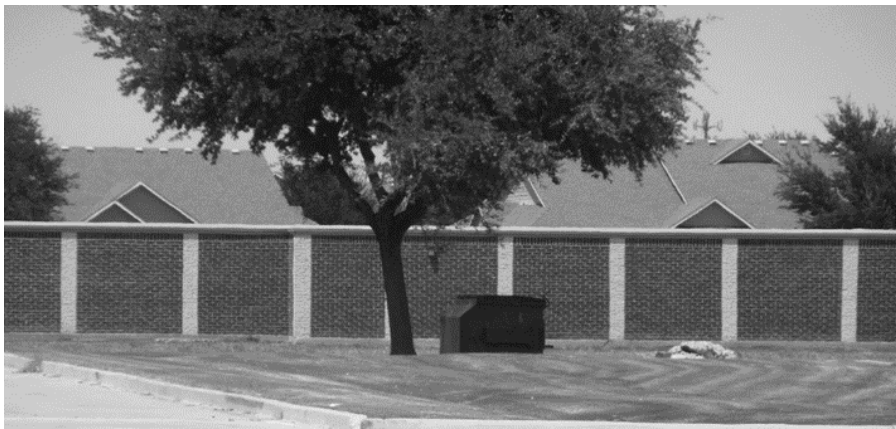
Eight (8) Foot Screening Masonry Wall
