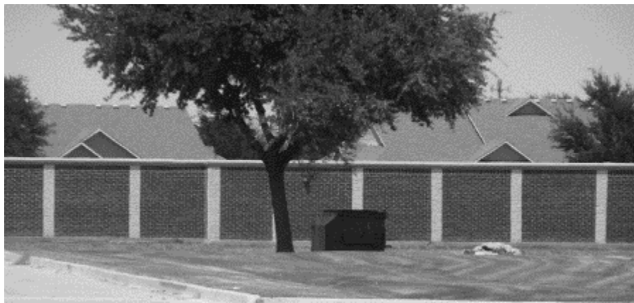
Eight (8) Foot Masonry Screening Wall
