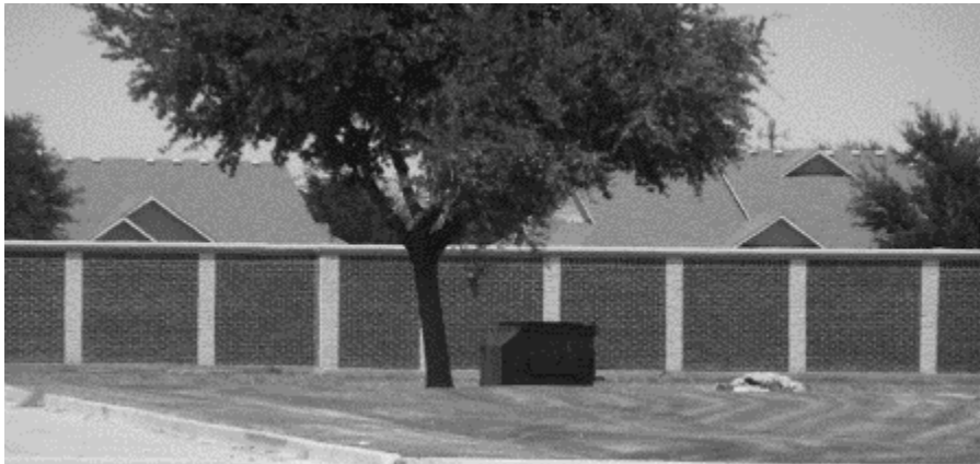
Eight (8) Foot Masonry Screening Wall
